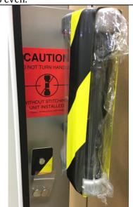
5.3) It is now safe to remove the safety tape. Cut the tape on both handles and discard. Remove the safety bolts (qty 2) using a 9/16" socket wrench and replace with the included beauty caps (pictured at right).
